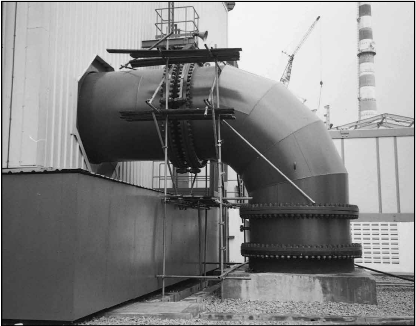
Mercer's Style 501 96" diameter expansion joint employed in a typical configuration in a Malaysian power plant.
